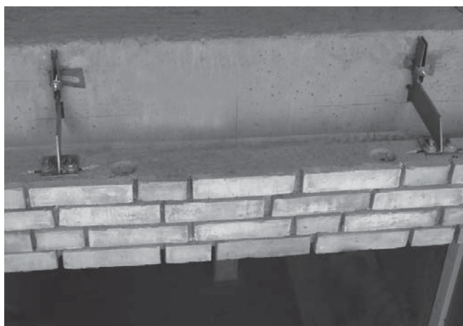
HK4-S with HTA-ES for pre-cast lintels
