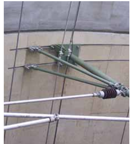
Connections to precast tunnel linings: Curved cast-in HALFEN channels allow accurate and clean installation of mechanical and electrical services, without dust and noise from drilling; damage to the concrete; or the power and access problems associated with welding.
