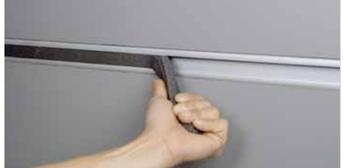
2. When the formwork is removed the foam filler strip is simply removed from the HALFEN channel.
