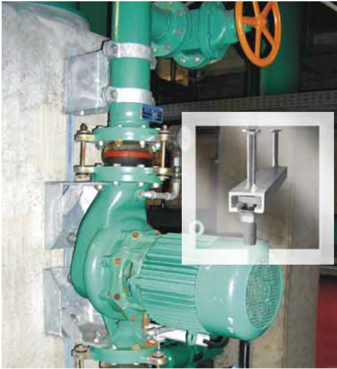
Equipment connections: HALFEN channels allow accurate and clean installation of plant and equipment. HALFEN toothed channels provide high load capacities while providing vertical adjustment.
