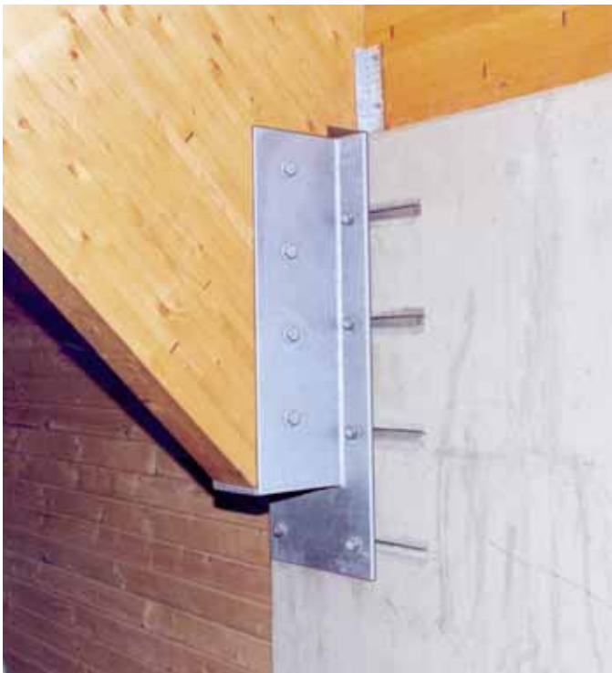
Roof and beam connections: HALFEN channels allow secure and accurate installation of major structural elements.
