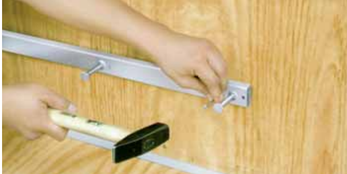
1. After marking the approximate position needed for connections, HALFEN channels are simply nailed to the formwork before pouring concrete.
