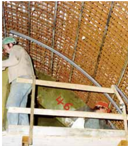
Connections to tunnel linings: Curved or straight cast-in HALFEN channels allow accurate and fast installation for lighting systems, ventilation equipment, and power delivery catenaries.
