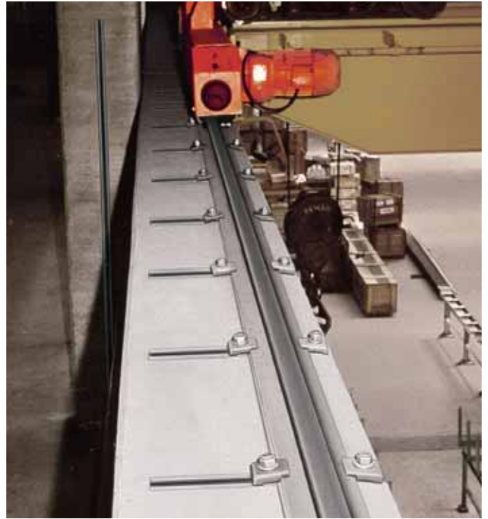
Craneway connections: HALFEN channels allow accurate alignment, and fast installation. HALFEN toothed channels provide high dynamic side load capacities.
