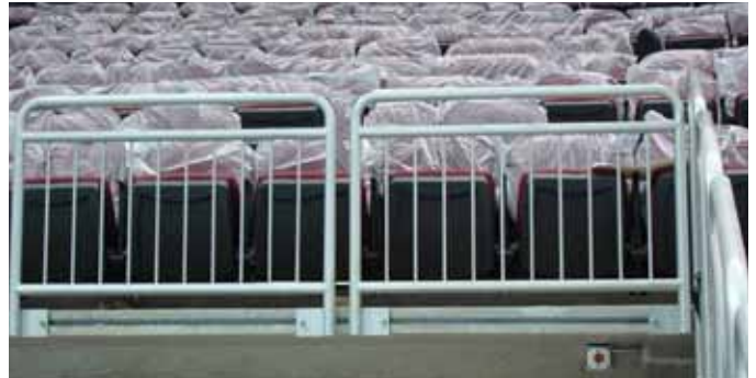
Handrail installation: HALFEN channels provide secure connections for high loads close to the edge of concrete, while allowing fast and easy installation adjustment. In stadiums handrails can be removed or re-positioned for disabled access or special crowd control.
