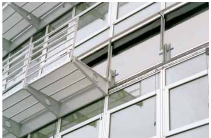
Walkway, window cleaning, and sunscreen connections: HALFEN channels in stainless steel or hot dip galvanized finish allow totally secure and accurate connections for building components requiring high levels of safety.
