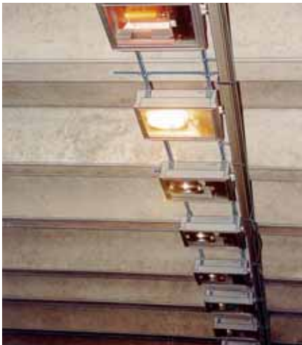
Connections in road tunnels: Cast-in HALFEN channels when used with HALFEN framing channels provide two-way tolerance for the accurate installation of lighting systems, and ventilation equipment. Channels made from special high corrosion resistance grades of stainless steel are available for conditions with high concentrations of sulphur dioxide or chlorides.
