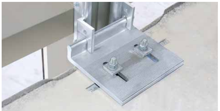
Curtain wall installation: Flush mounted HALFEN channels embedded in concrete enable rapid and accurate façade installation. This allows the building to be quickly enclosed aiding the programme for the completion of interior finishes.
