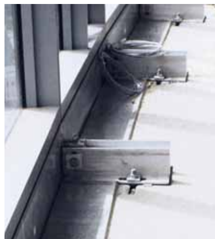
HALFEN channels embedded in concrete form the basis of adjustable façade attachment.
