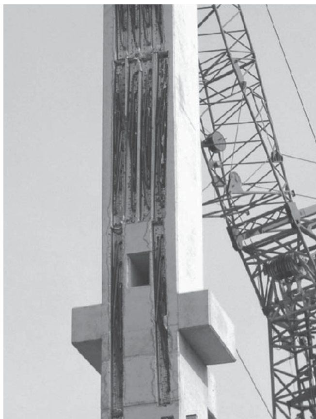
Connection; column — wall
