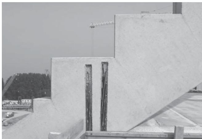
Connection; grandstand in stadium — supporting element
