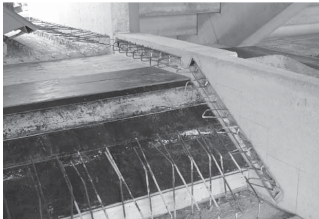
Connection; wall — Stair landing
