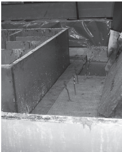
Installation at the precast plant: SPA-A
